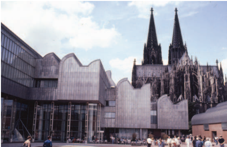
Figure 4.56: Stainless steel façade reflecting the roof form of the polar-oriented skylight system at the Wallraf-Rickartz Museum
