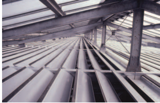
Figure 4.30: Underside of the roof glazing and upper surface of the motorized light control louvres at the Staatsgalerie
