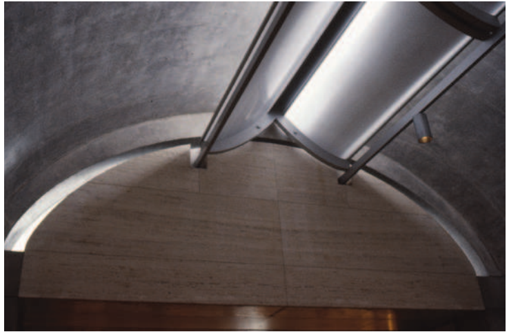
Figure 4.98: Detail of the ceiling vaults separated from the walls by a glass strip, giving the appearance of floating, at the Kimbell Art Museum
