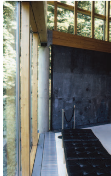
Figure 4.104: One of the heavy security panels at the Burrell Collection that has failed to retract below floor level
