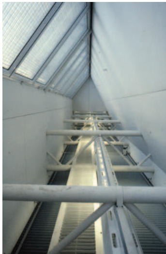
Figure 4.63: Skylights and fluorescent lighting at the Waikato Art Museum, with louvres below that are adjusted for seasonal variation of daylight availability
