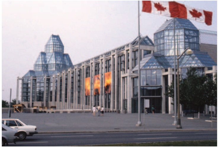
Figure 8.5: The National Gallery of Canada, Ottawa, with the entrance at the near corner and the Grand Hall at the far end
